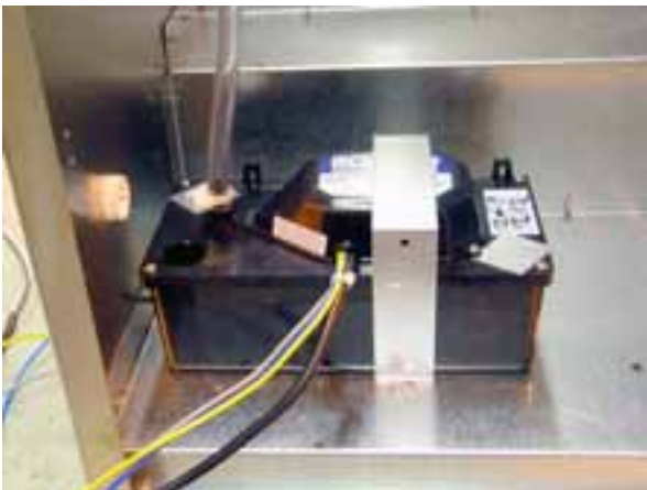
Figure 6: Condensate pump
