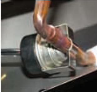
Figure 4: Defrost thermostat
